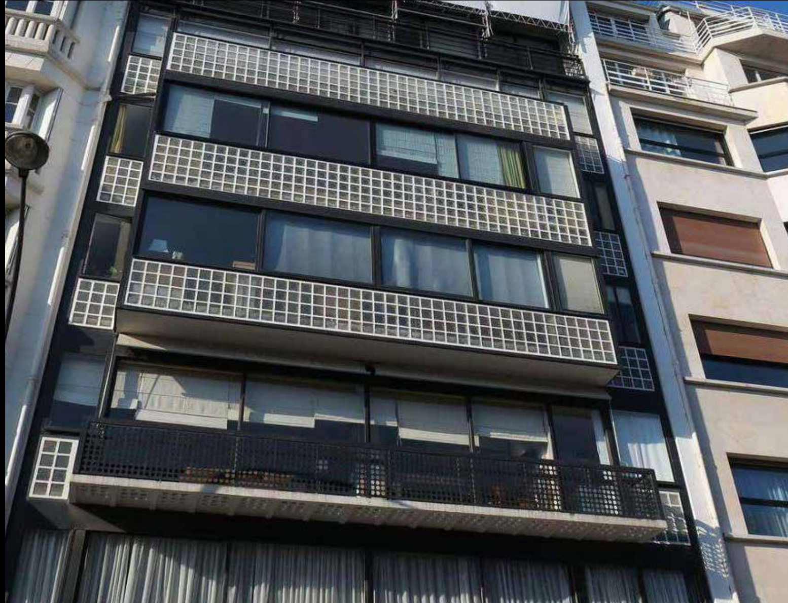
Appartement Molitor - Paris - 1934
